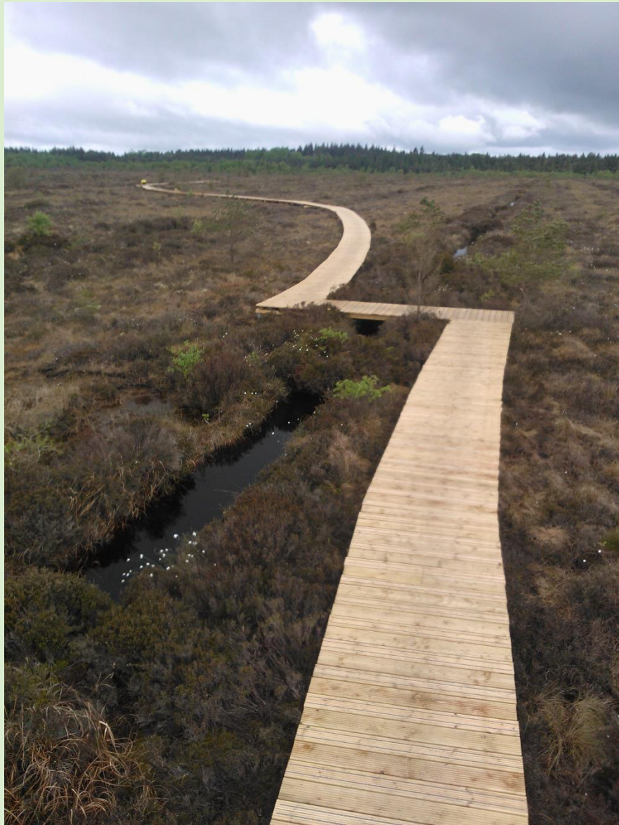
Photograph 2: Section of the finished Boardwalk across high bog (Source Chris Uys)
